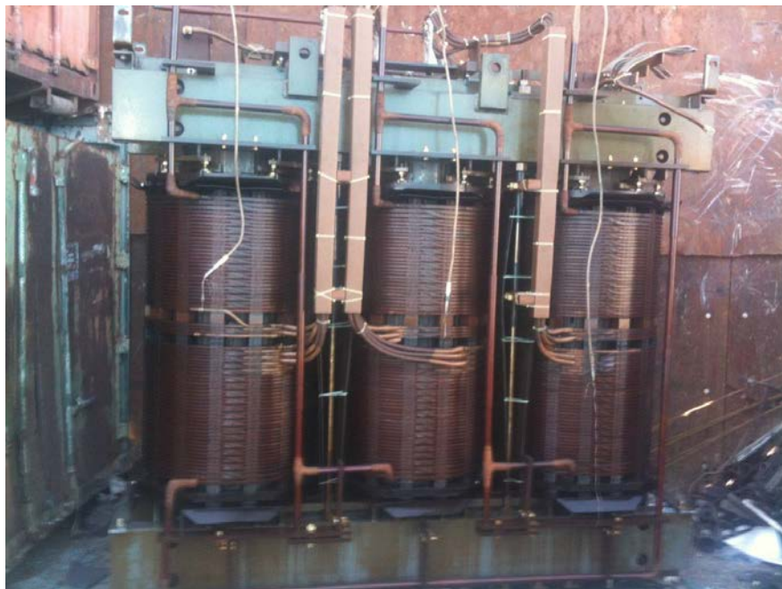
Cores and Windings
